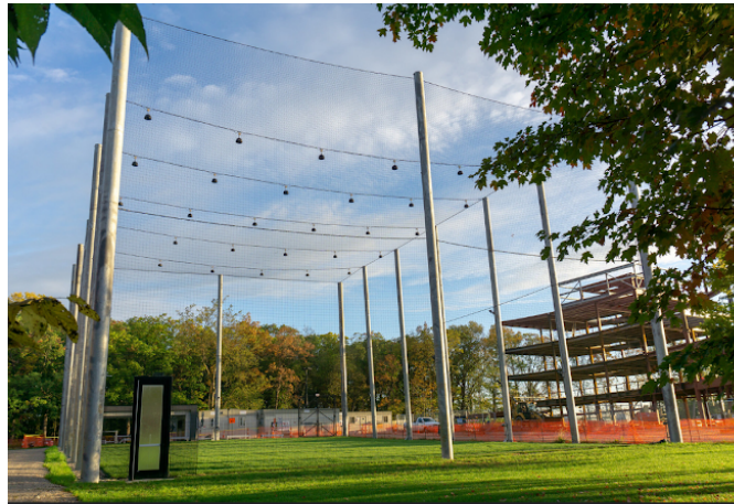
Figure 5. M-Air Outdoor Flight Facility
